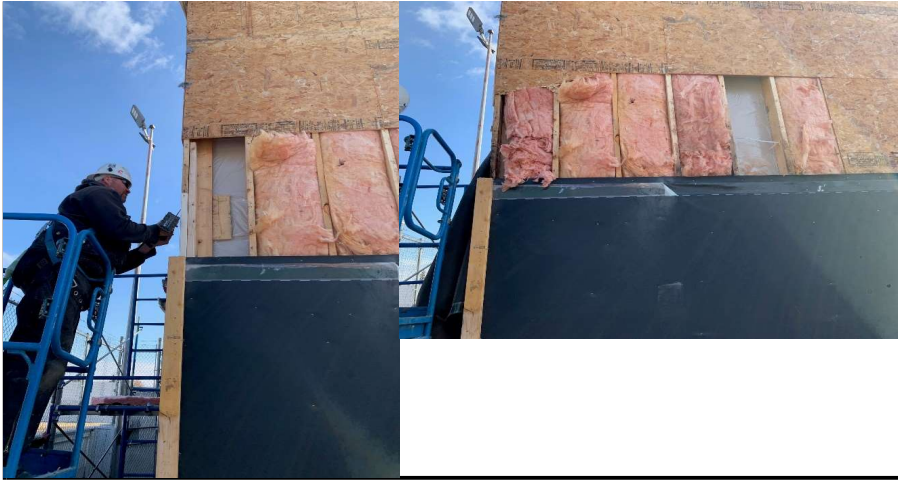
West Wall repair, insulation removed new insulation installed.
