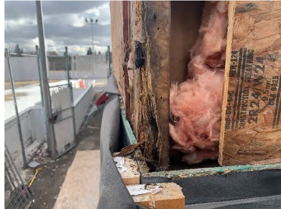
Photograph 2 Wood rot of corner stud framing along the upper northwest elevation.
