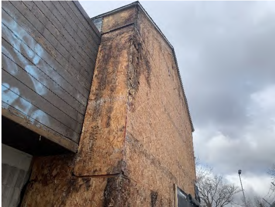
Photograph 1 Deteriorated OSB sheathing on the north elevation.
