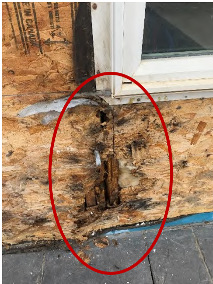
Photograph 3 Deteriorated and rotten stud members at the centre window on the west elevation.
